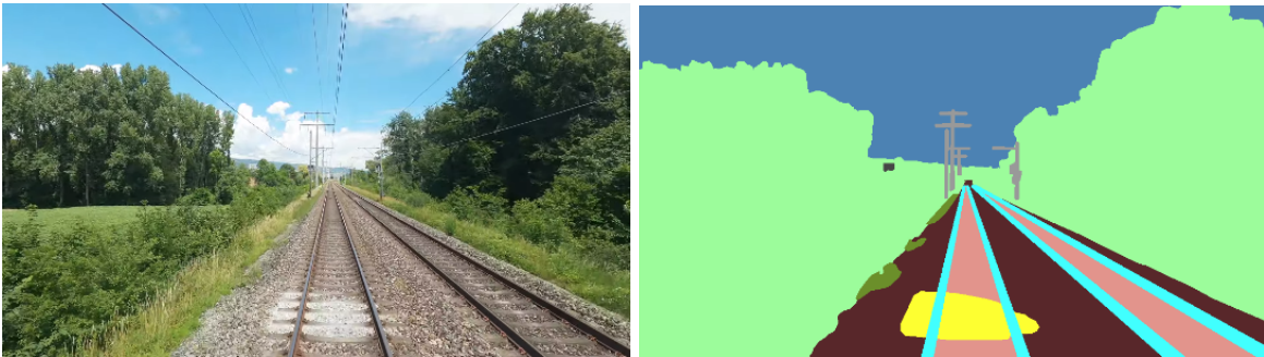
(b) Mud Pumping marked in yellow
